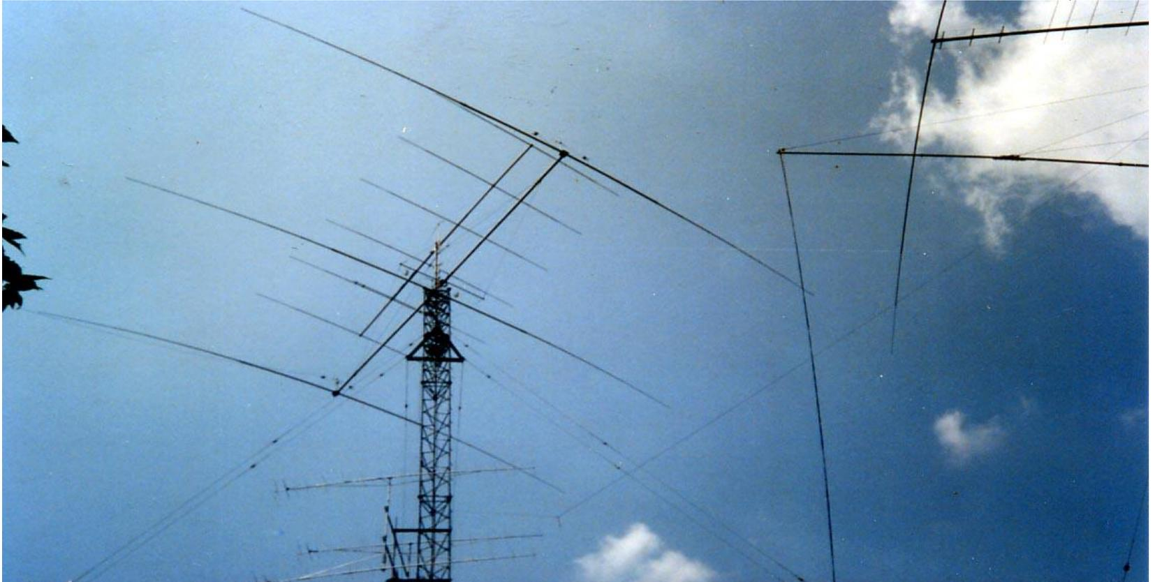
K3ZO's very successful horizontally polarized 3 element Yagi changed my thinking about 80 meter antennas for DX
